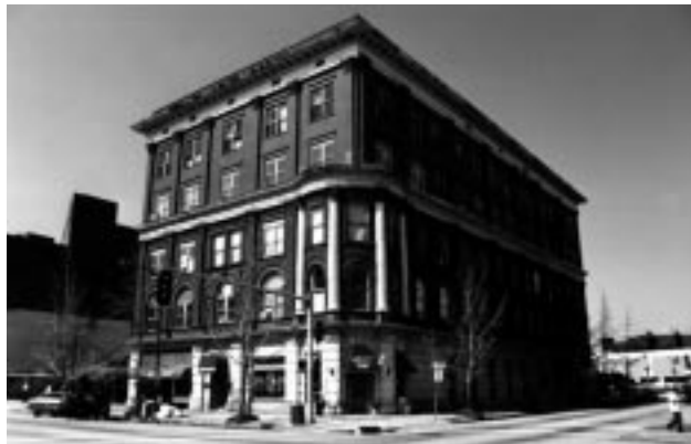
The retention of original materials (brick, rusticated stone, intact windows) could make the rehabilitation of this 1896 building a very successful project.
