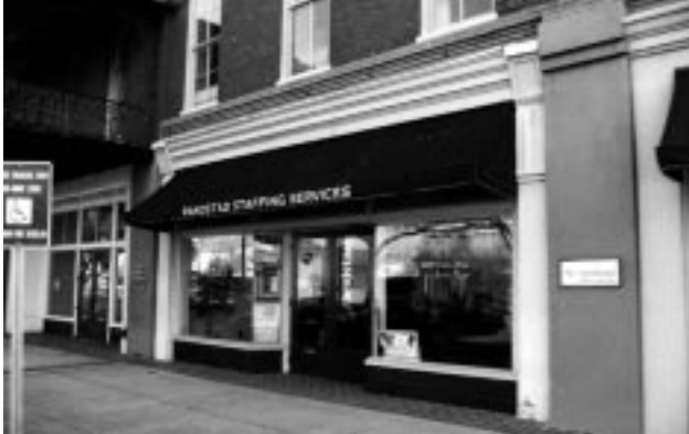
Good example of an intact recessed entrance.
