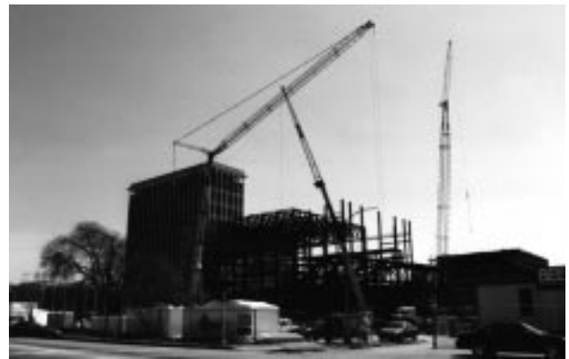
New construction for the River Center for the Performing Arts.
