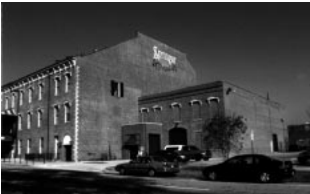
The addition to the side of the historic Spring Opera House suggests, without replicating, the design characteristics of the windows as well as the brick material of the original building. This addition does not overpower or detract from the historic opera house.
