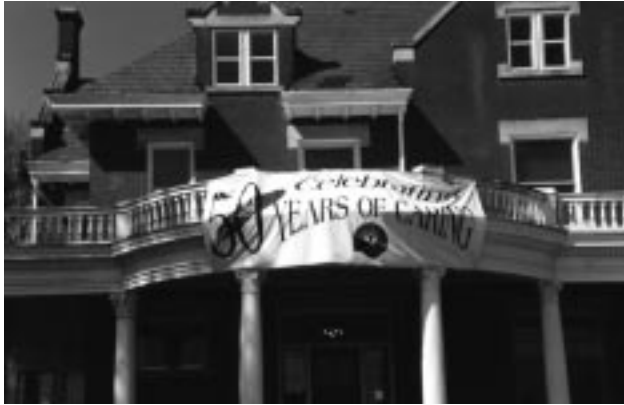
Inappropriate example of a temporary banner sign.
