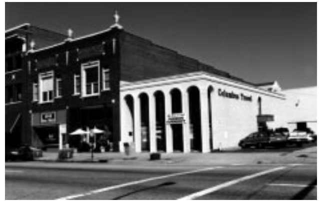
This building's tall arches and light-colored brick exterior does not respect the existing look of the historic streetscape.
