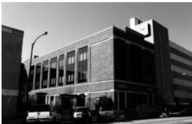
Good example of infill construction that respects the dominant setback, common materials, and height of many downtown commercial buildings.
