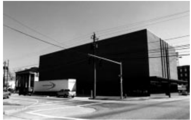
An example of extremely inappropriate new construction; the building's solid brick mass dwarfs the antebellum frame house to the far left.
