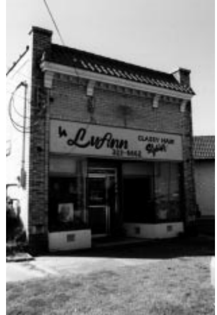
This small commercial building has retained its original clay tile roof and recessed entrance.
