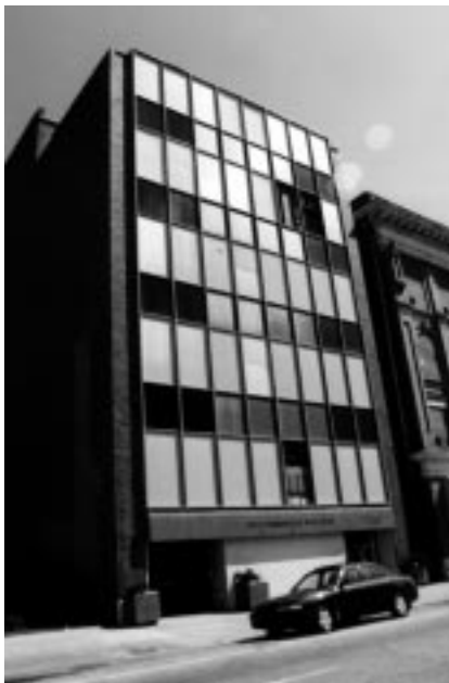
This c1960s façade is covering the original façade.
