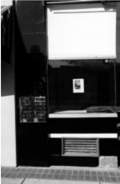
The original brick storefront of this building is still intact beneath the nonhistoric enamel panels.
