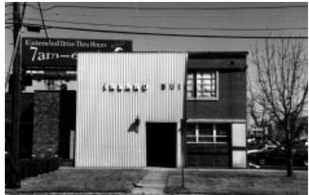
Brick façade requiring attention.
