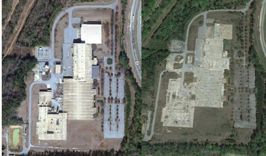
The Swift Denim Plant at the time of closure (left), the demolished site (right)
