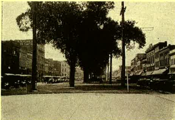
Broad Street. The trees still stand on this portion of the wide street although taken over by business. Compare with next photograph
