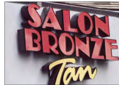
Internally-lit plastic-front channel letters.
