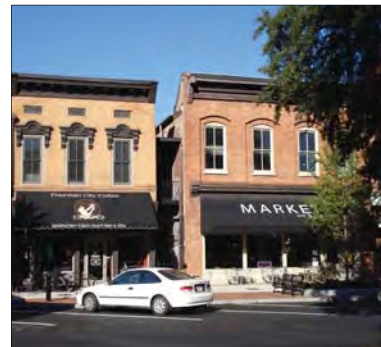
Typical 2-story historic commercial buildings in downtown Columbus.
