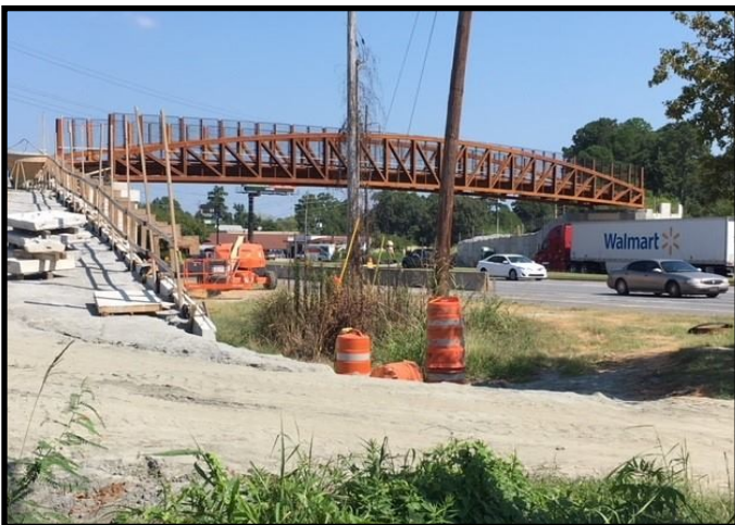
Follow Me Trail Bridge being installed
