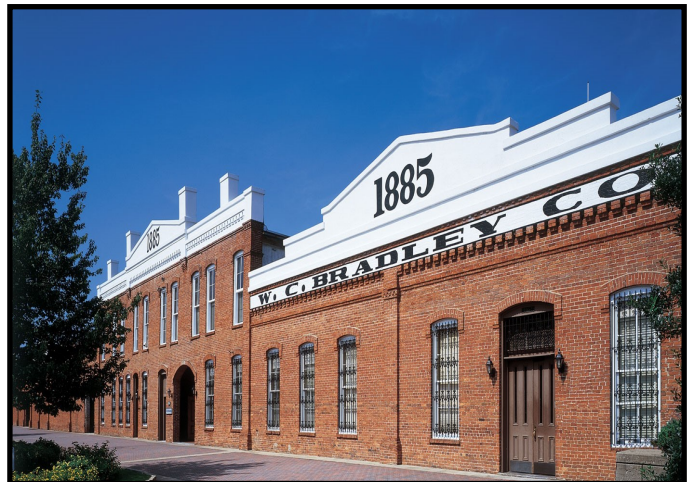
W.C. Bradley Co. Building
