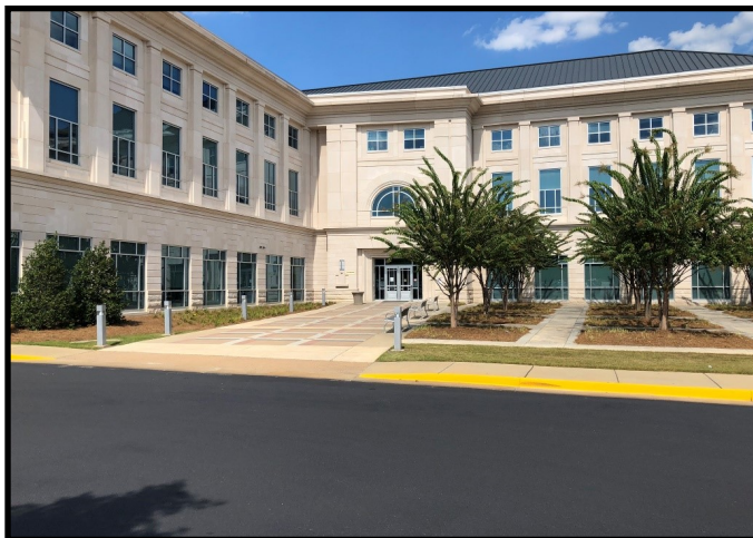
Muscogee County School District Admin. Building
