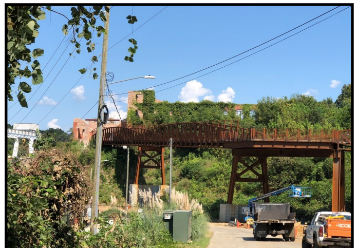
River Walk Bridge Expansion
