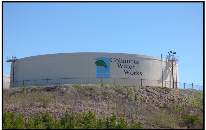
Columbus Water Works Treatment Facility
