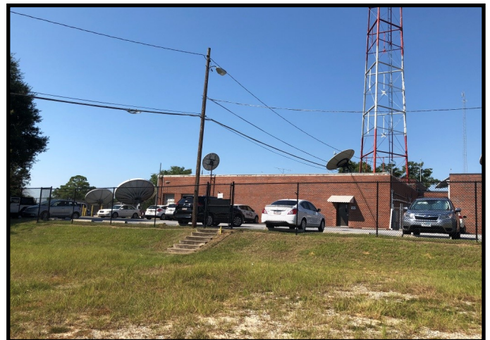
WRBL Station and Broadcast Tower
