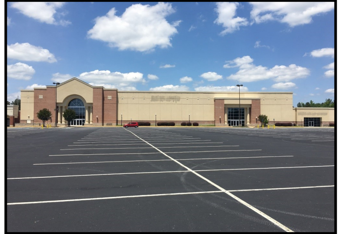
Vacant Sears Building
