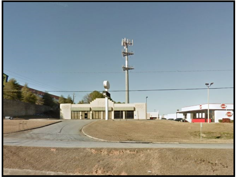
Cell Phone Tower along Manchester Expressway
