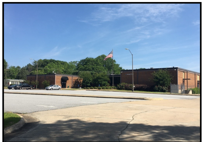
Georgia Power Office on Gentian Road
