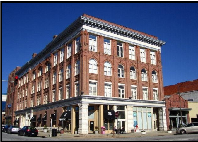
Traditional storefronts with living space above
