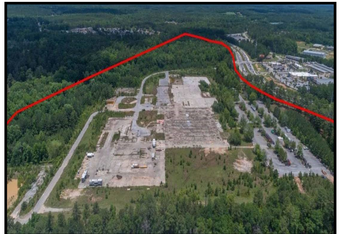
Swift Spinning Mills Site Aerial
