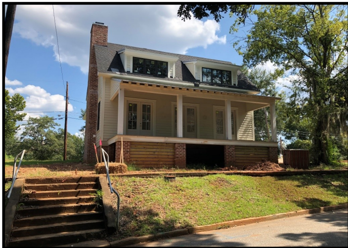
New single family housing under construction
