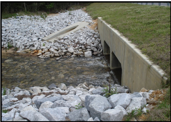
Lindsey Creek passing through a culvert
