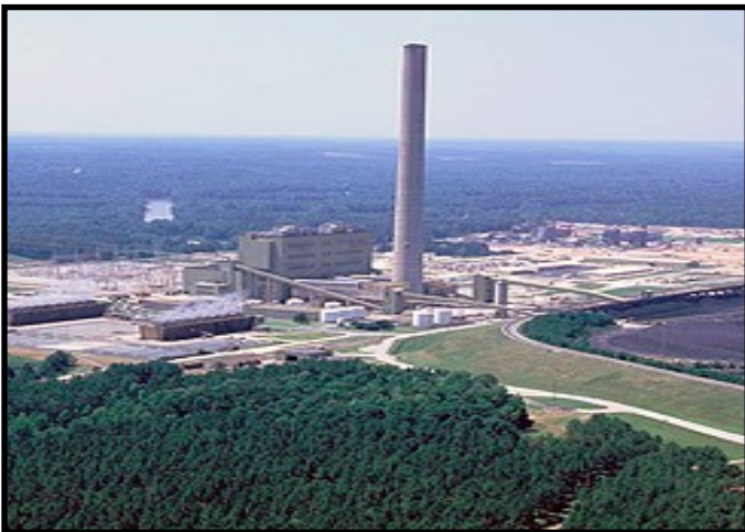
Plant Wansley, a coal and natural gas facility approximately 75 miles north of Columbus.
