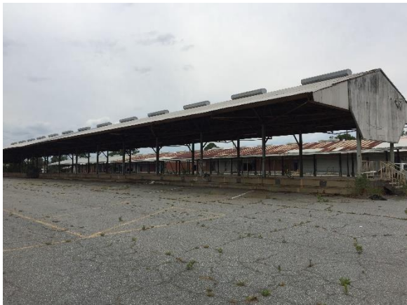
Photo #39 View (south side) of Loading Area #1 (Building 9).
