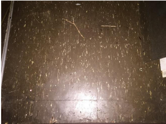
Photo #7 Example view of asbestos-containing 12x12 brown VCT & black mastic in office area, Warehouse #1 (Building 1).
