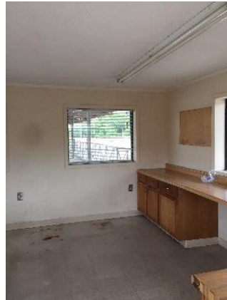
Photo #38 Interior view of office at west end of Loading Area # 2 (Building 8).
