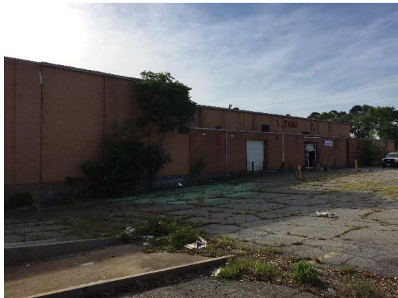
Photo #21 View (west side) of Warehouse #4 (Building 4).
