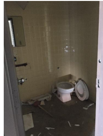
Photo #20 Example view of bathroom in vendor area w/ asbestos-containing ceramic wall tile mortar, Warehouse #3 (Building 3).
