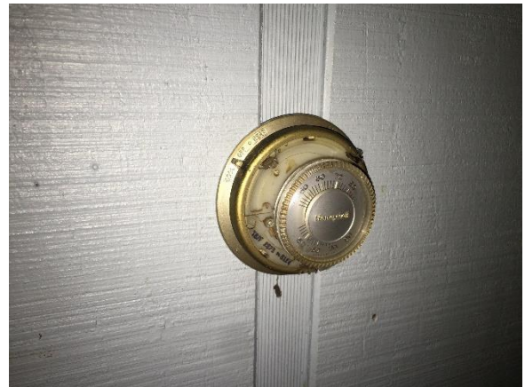
Photo #46 Example view of mercury-containing thermostat in office area, Warehouse #1 (Building 1).
