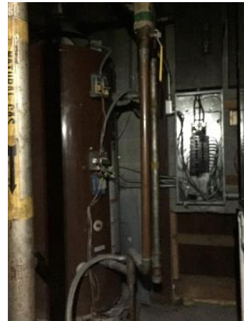
Photo #44 View of mechanical closet in restaurant (Building 10).
