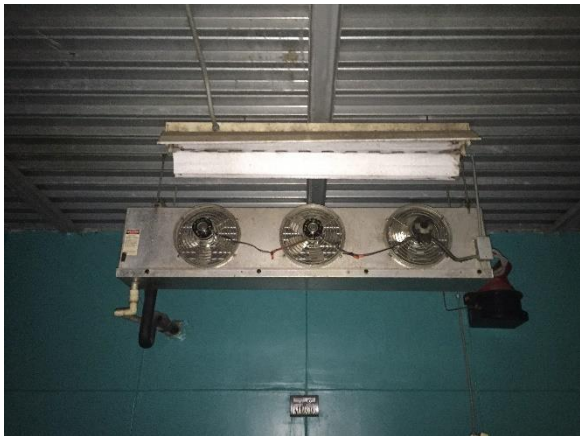
Photo #45 Example view of cooling unit in walk-in cold storage units in site buildings.
