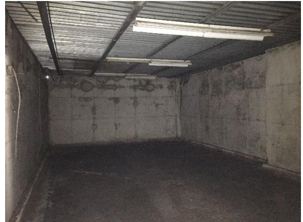
Photo #14 Example view of walk-in cold storage unit w/ asbestos-containing insulation panels in Warehouse #2 (Building 2).
