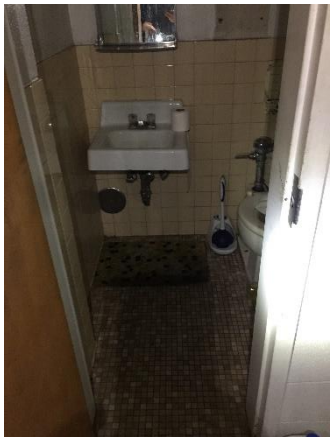
Photo #29 Example view of bathroom w/ asbestos-containing ceramic wall tile mortar, office area, Warehouse #4 (Building 4).
