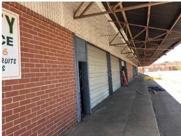
Photo #11 Example view of front loading area (south side) of Warehouse #2 (Building 2).
