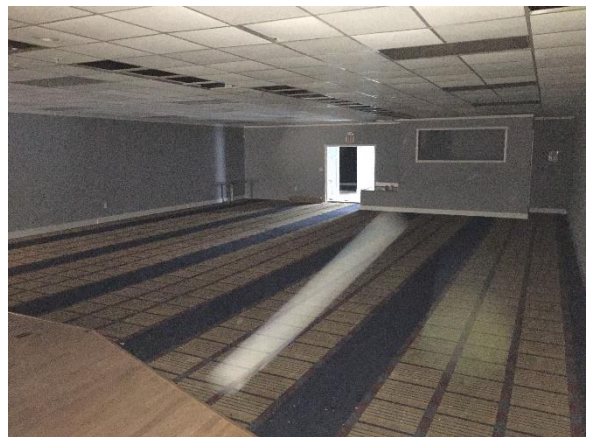
Photo #42 Example view of dining area of restaurant (Building 10).
