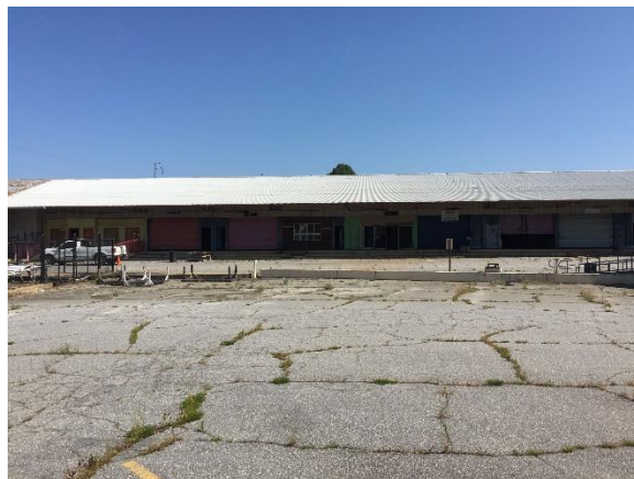
Photo #2 View (south side) of Warehouse #1 (Building 1).
