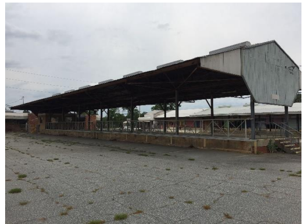
Photo #36 View (south side) of Loading Area #2 (Building 8).
