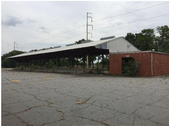
Photo #33 View (north side) of Loading Area #4 (Building 6) and bathroom at west end.
