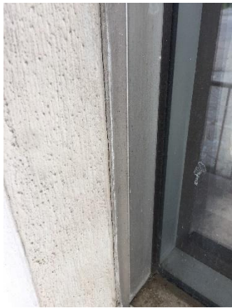
Photo #9 Example view of asbestos-containing exterior door caulk associated with the office area, Warehouse #1 (Building 1).
