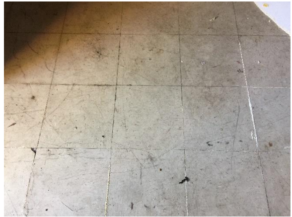
Photo #8 Example view of 12x12 white VCT & asbestos-containing black mastic in office area, Warehouse #1 (Building 1).
