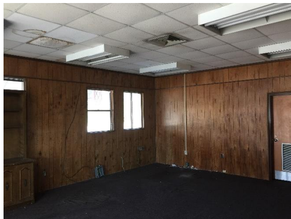
Photo #4 Example view of office area interior, Warehouse #1 (Building 1).
