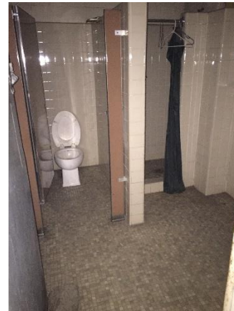
Photo #32 Example view of bathroom w/ asbestos-containing ceramic wall tile mortar, former Columbus Towing & Recovery (Building 5).
