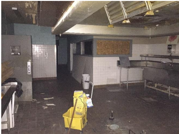
Photo #43 Example view of kitchen area of restaurant (Building 10).
