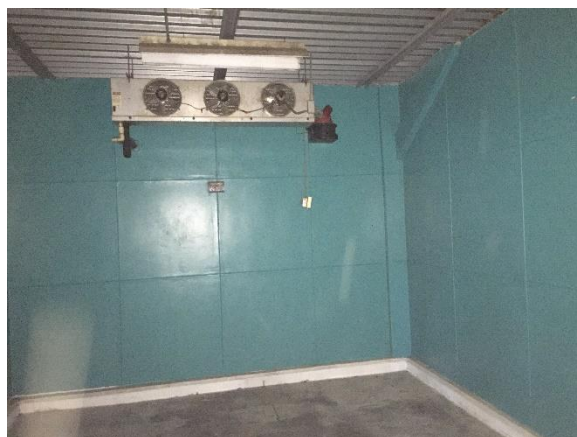
Photo #6 Example view of walk-in cold storage unit interior w/ asbestos-containing insulation panels, Warehouse #1 (Building1).
