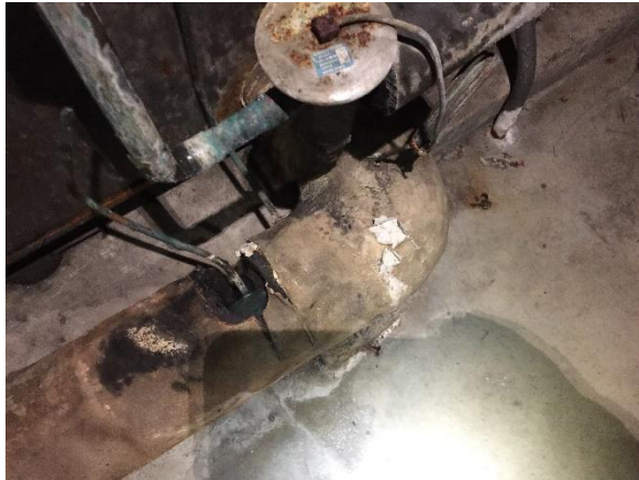
Photo #27 Example view of asbestos-containing mudded thermal pipe insulation, office area mechanical room, Warehouse #4 (Building 4).
