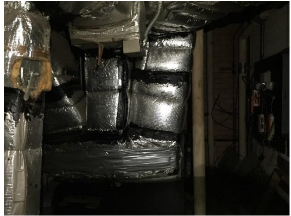
Photo #28 Example view of asbestos-containing tar coating on foil HVAC insulation, office area mechanical room, Warehouse #4 (Building 4).
