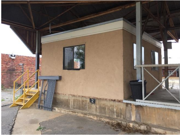
Photo #37 View of office at west end of Loading Area # 2 (Building 8).
