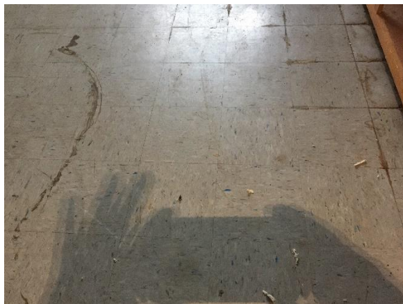
Photo #23 Example view of 12x12 blue-speckled VCT w/ asbestos-containing black mastic, office area, Warehouse #4 (Building 4).
