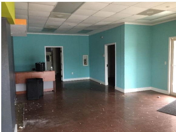
Photo #41 Example view of entrance/lobby area of restaurant (Building 10).
