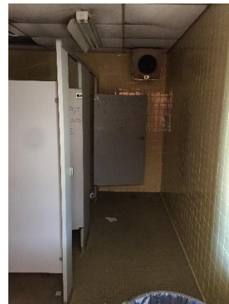
Photo #12 Example view of bathroom at west end of Warehouse #2 (Building 2) w/ asbestos-containing ceramic wall tile mortar.
