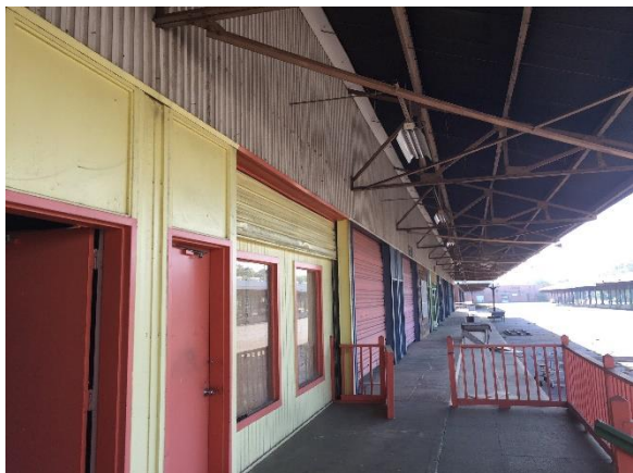
Photo #3 Example view of front loading area (south side) of Warehouse #1 (Building 1).
