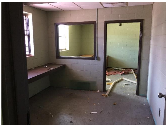
Photo #17 Example view of vendor area office w/ asbestos-containing 2x2 ceiling tile, Warehouse #3 (Building 3).
