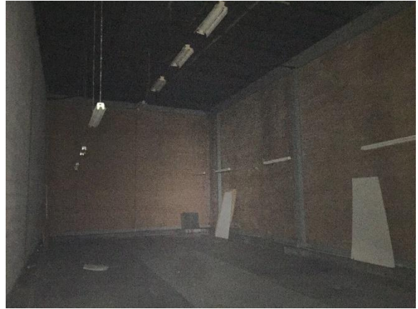
Photo #26 Example view walk-in cold storage w/ asbestos-containing insulation panels, Warehouse #4 (Building 4).
