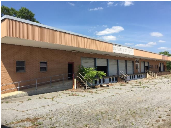
Photo #15 View (south side) of Warehouse #3 (Building 3).
