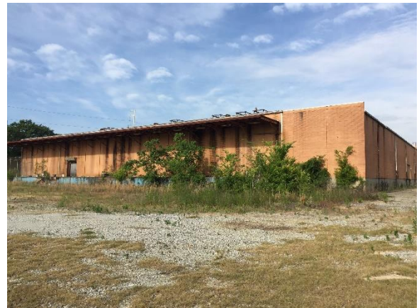
Photo #22 View (east side) of Warehouse #4 (Building 4).
