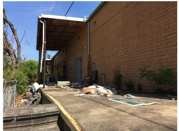
Photo #16 Example view of loading dock (north side), Warehouse #3 (Building 3).
