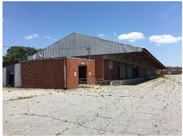
Photo #10 View of Warehouse #2 (Building 2), west end w/ bathrooms.
