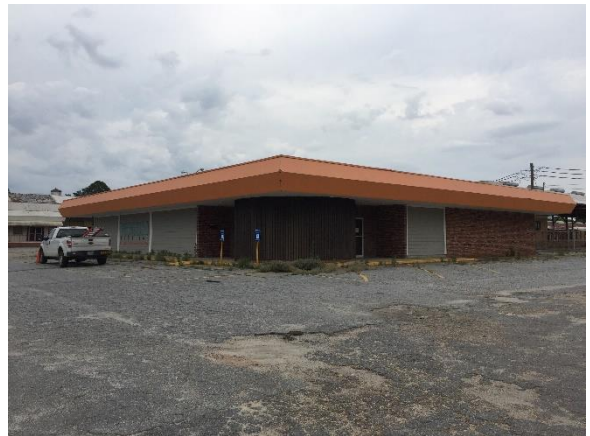
Photo #40 View (south & west sides) of restaurant (Building 10).
