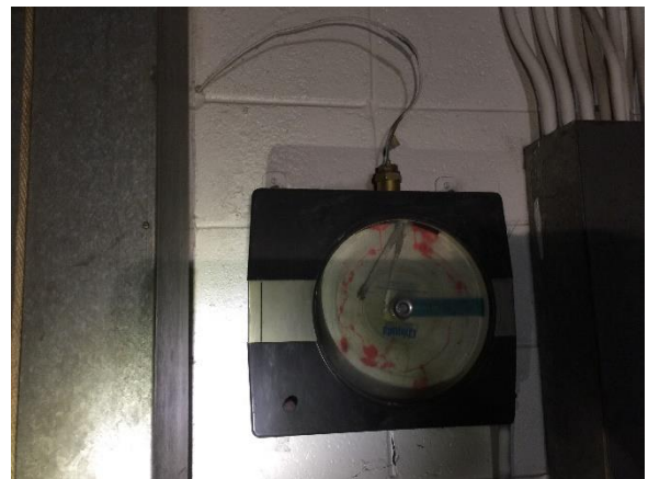
Photo #48 View of mercury-containing thermometer in Warehouse #4 (Building 4).
