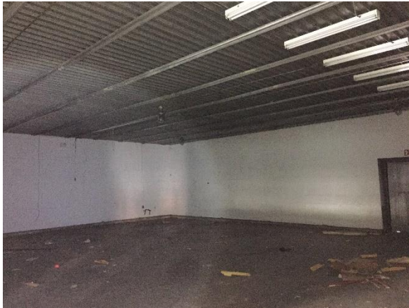
Photo #19 Example view of walk-in cold storage unit w/ asbestos-containing insulation panels, Warehouse #3 (Building 3).
