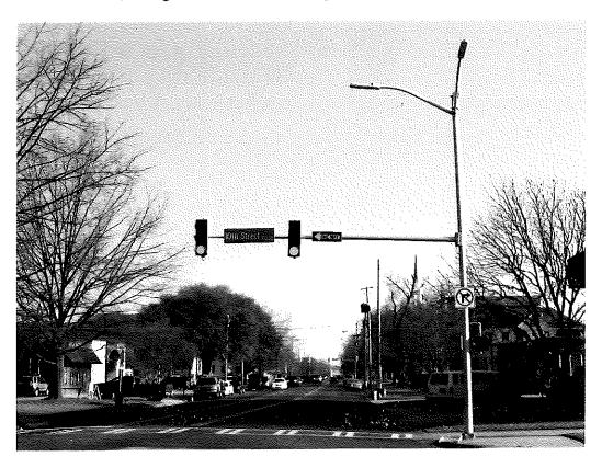
Example – Standard DOT Steel Mast Arm Strain Pole
